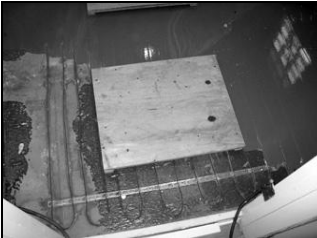
Figure 2: Self-leveling mortar being applied over the floor heating cable.
